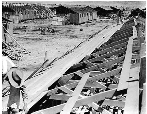
Poston, Arizona, center under construction.
