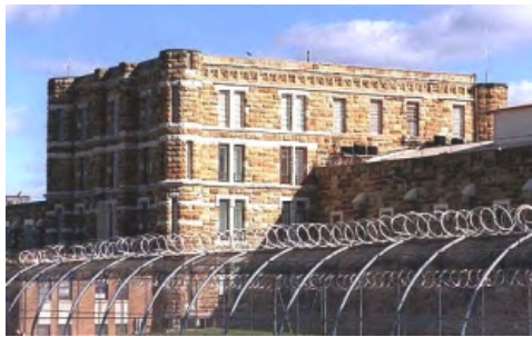
Lansing Correctional Facility. The injection chamber is the corner room on the top floor.
